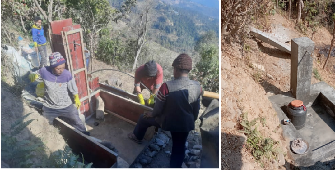
Photograph 1: Construction of water taps in Badarpa
